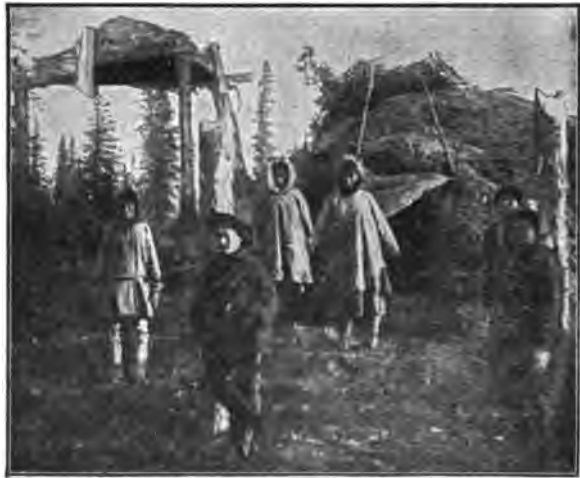
Native Igloo, with Scaffold for Stores.
